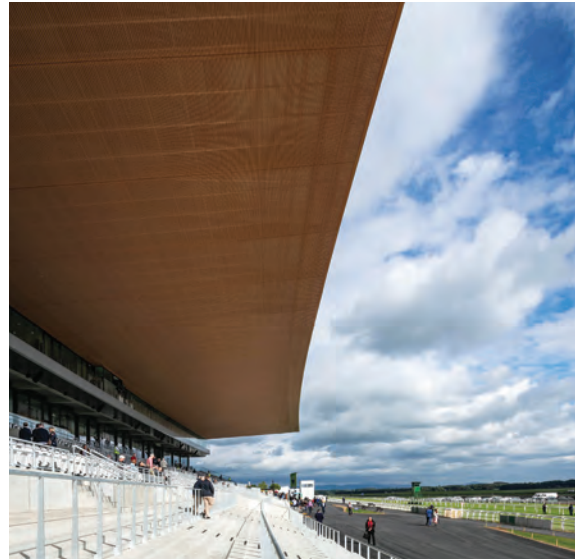
Above: The complex roof design involved careful coordination with the facade
